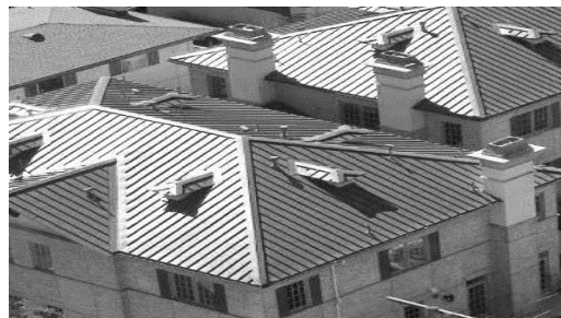
Figure 2: Galvanized roofing sheets
